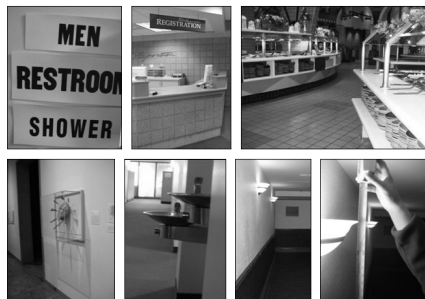
All elements: signage, counters, water fountains, protruding objects, etc.
